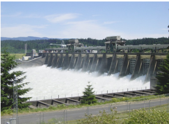
Hydroelectric Dam. Photo Credit: Kristin Manke & Richard May/Flickr
